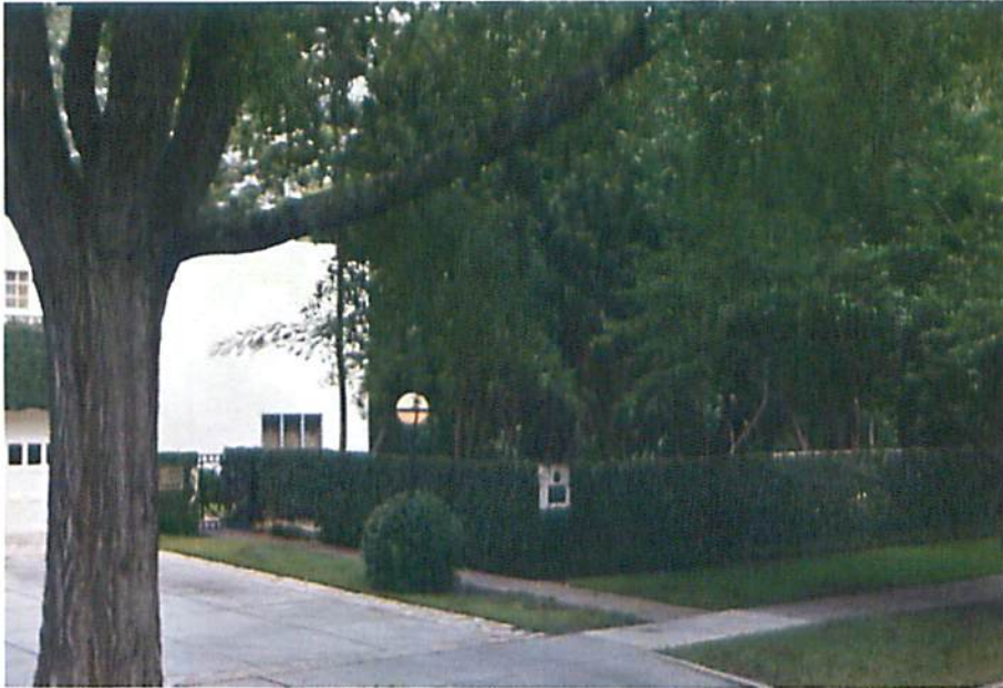
Existing wall, covered with vegetation
