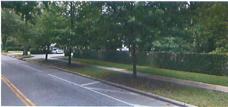
Existing wall, looking south
